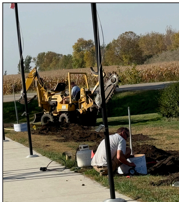
Crews from G&R Electric did trenching work prior to the installation of new outdoor light fixtures.
