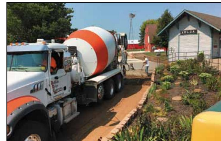
A new concrete pathway was poured last summer and fall, between the Helmberger building and the Moline General Store. Photo shows a Doug Kass Construction crew smoothing a pour near the depot.
